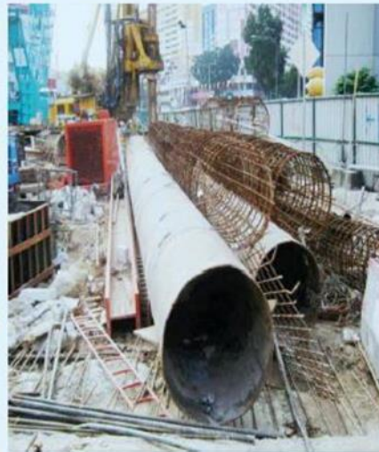
Improper placement and storage of materials
