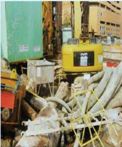
Improper placement and storage of materials
