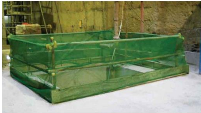
Railings used to fence off hazardous areas must be at least 1.1 m tall
