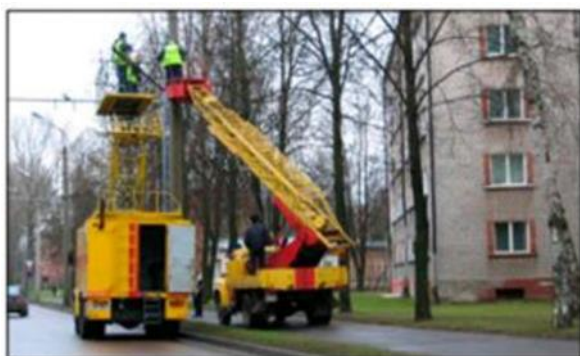
Work area of an aerial lift not fenced off
