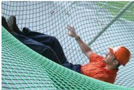
Fall protection net or stable and secure railings
