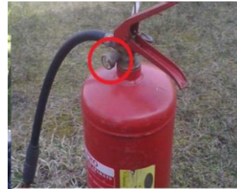
The pressure gauge of the fire extinguisher is damaged and the information about the certification period and performed inspections is damaged and illegible
