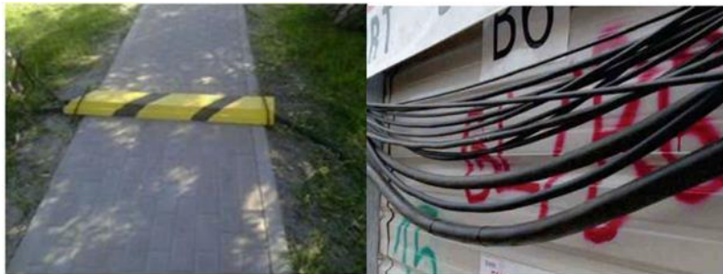
Covered or elevated cables in traffic areas
