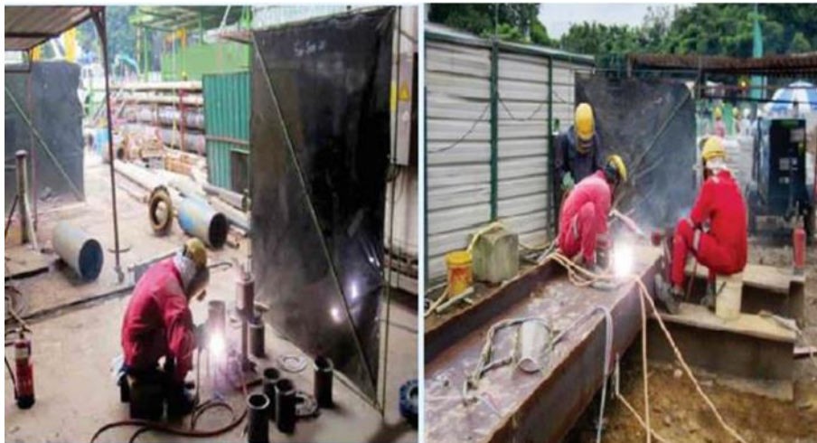
A portable curtain or protective wall is installed at the welding area to protect workers against exposure to ultraviolet radiation
