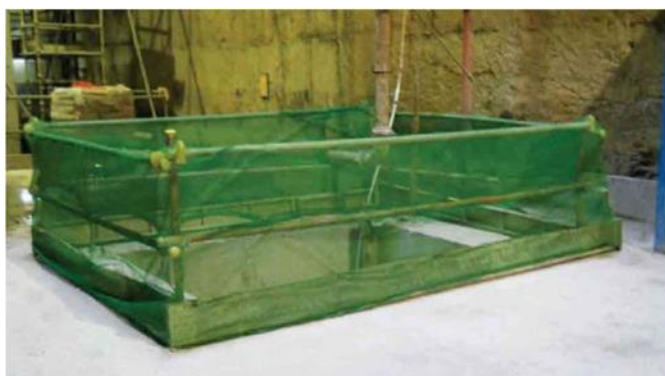
Railings used to fence off hazardous areas must be at least 1.1 m tall
